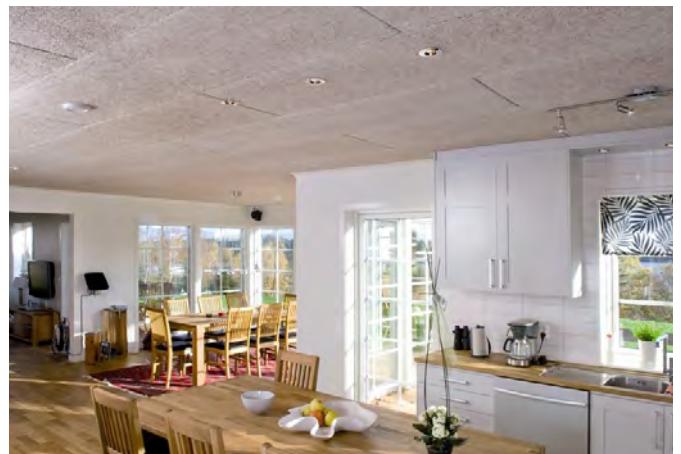
Figure 1 (L) A wood-wool cement board with ingredients like spruce wood-wool, cement, water and waterglass. (R) Wood-wool cement boards applied on ceiling for sound absorption.
