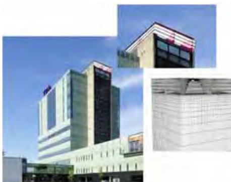
Figure 5: Wind energy roof on Vertigo building (Ferraro and Moonen, 2011)
