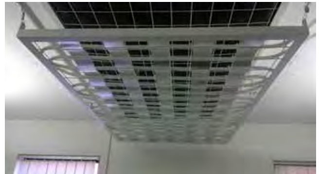
Figure 6: Radiant Ceiling with the metal slabs
